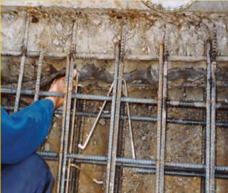
SLOWLY PRESS ON TO CONNECTING SLAB JOINT.
