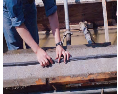
CONNECT TWO PIECES BY END-BUTT JOINING.
