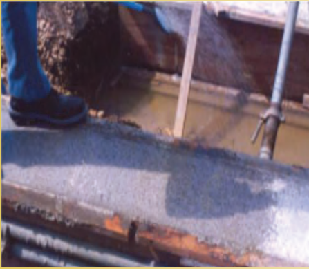
BRUSH OFF DIRT AND WET CONCRETE JOINT.
